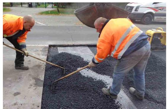
Pic. 9: HMA application over ADFORS GlasGrid PG
