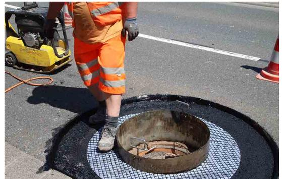
**Abb. 4:** ADFORS GlasGrid PG installation for manhole repair
