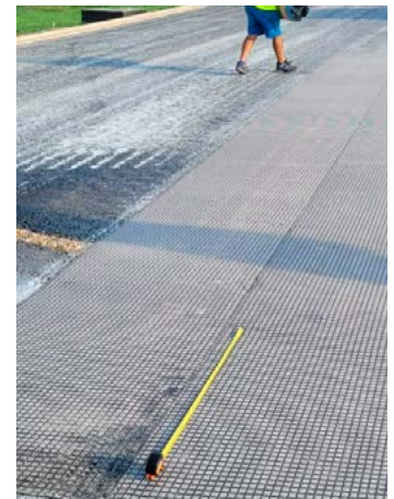
Installation of ADFORS GlasGrid Rapid Grid on a new highway, 2024
