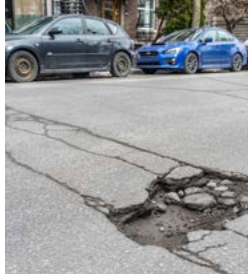
Example of cracking for local repairs
