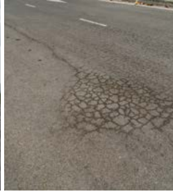
Example of cracking for area-wide repairs
