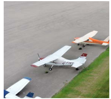
State of the pavement after 20 years in service (photo May 2018)
