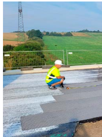
Installation of ADFORS GlasGrid Rapid Grid on a new highway, 2024
