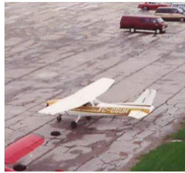
State of the pavement before the repair in 1992 safety compromised
