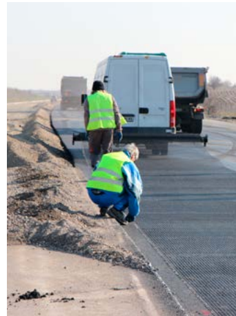
Installation of self-adhesive ADFORS GlasGrid GG 100 on A1 Highway Chirpan – Stara Zagora, 2021
