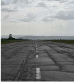
Example of cracking for area-wide repairs
