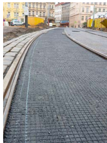
Installation of ADFORS GlasGrid Mastic, 2013
