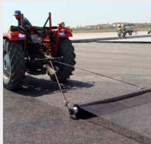
Installation of ADFORS GlasGrid at Atatürk Airport, 2010
