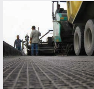
Installation of ADFORS GlasGrid at Atatürk Airport, 2010
