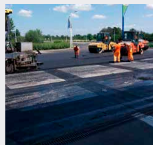
Installation of ADFORS GlasGrid in Belgrade, 2018
