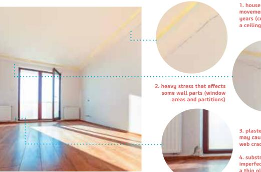
1. house settling – movements in the first years (corners between a ceiling and a wall)
