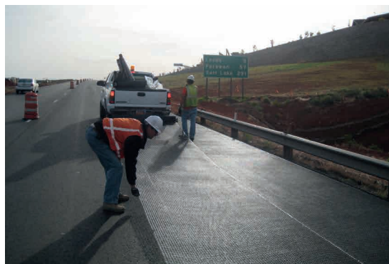
Pic. 4: Installation manuelle du ADFORS GlasGrid
