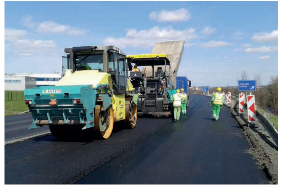
Pic. 9: Pave Overlay
