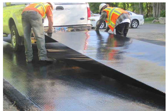
Pic. 2: ADFORS GlasGrid TF installation
