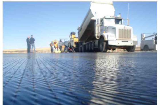
Pic. 1: ADFORS GlasGrid TF detail with film to bond layers
